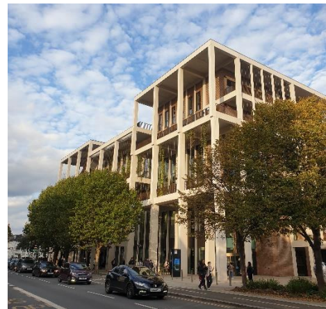
Bibliothek am Penrhyn Road Campus
