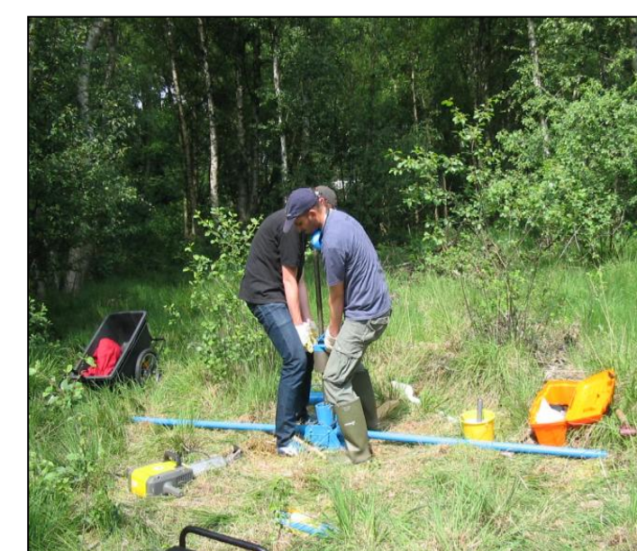
Fig 5a: Construction of a monitoring well
