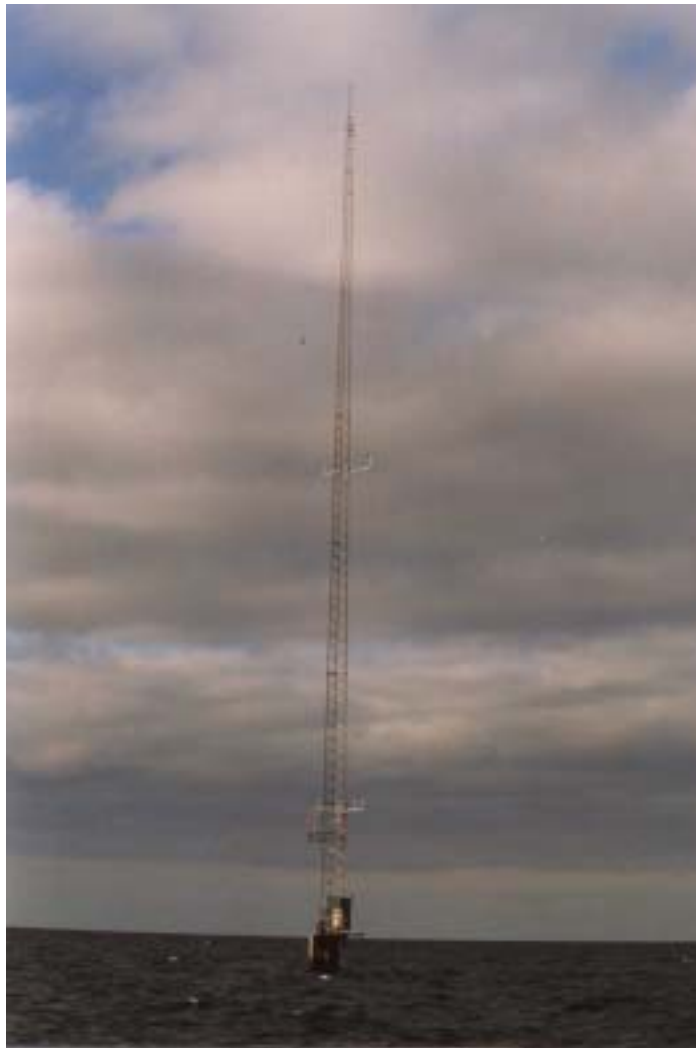
Figure 4: The meteorological mast of the Rødsand field measurement
