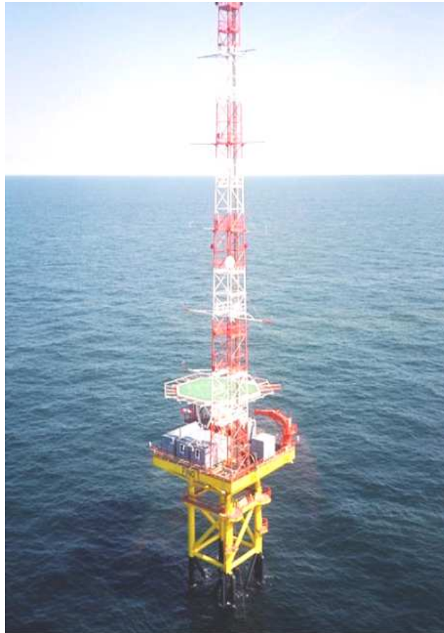
Figure 5.2: FINO measurement platform in the northern sea, from Germanischer Lloyd WindEnergie GmbH.
