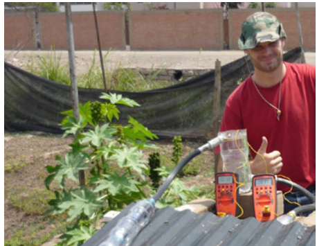
Manfred at his locally produced water heating system
