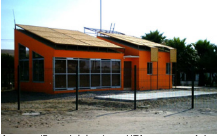
A new 'Energielabor' at UTA-campus, Arica, Chile
