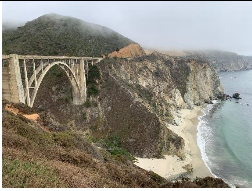
Bixby Bridge, Highway 1
