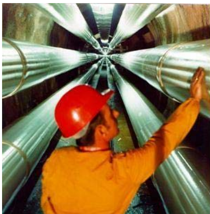
Figure 5 Example for tunnel laid GIL. Source: Siemens AG
